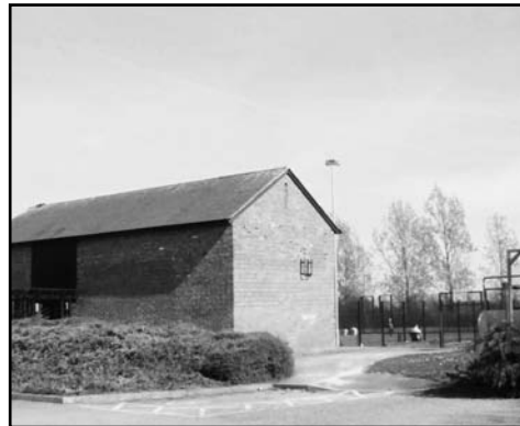
Downs Barn Pavilion. Picture: David Stabler
